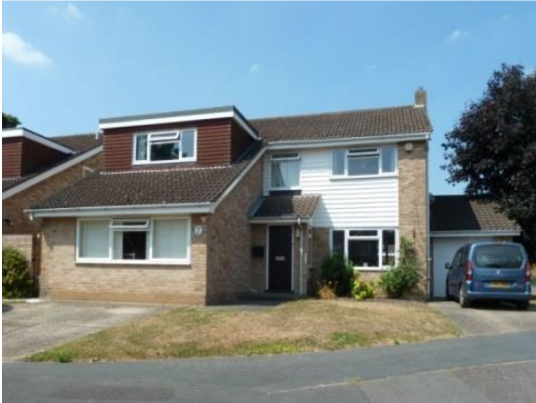
7 Grangewood, Wexham, Buckinghamshire, SL3 6LP OS Reference – SU 99349 81828 GPS – Lat – 51.526583 Long – 0.56925
